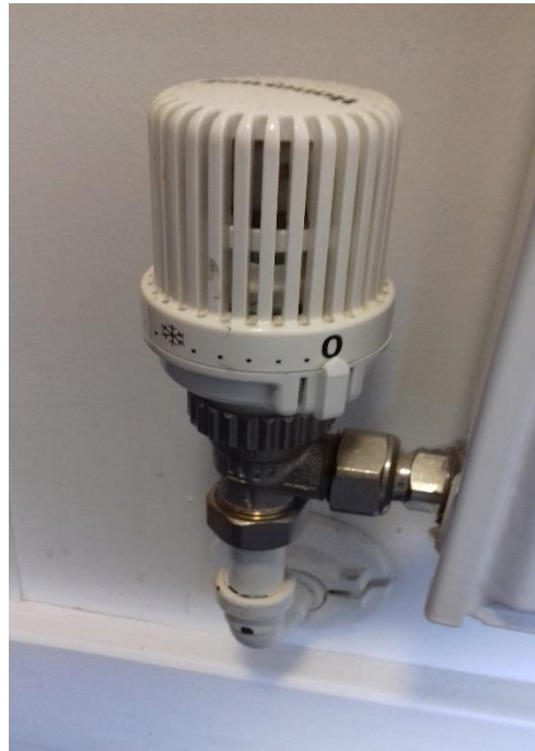
Figure 6 – TRV Off Position
