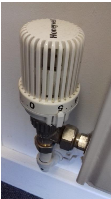
Figure 7 - TRV Maximum Setting
