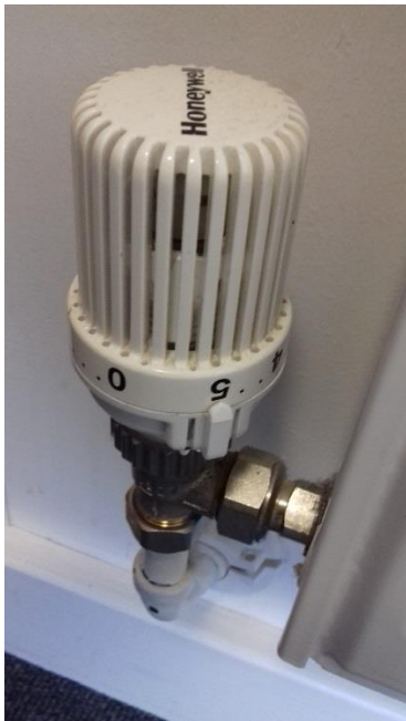
Figure 10 - TRV Maximum Setting
