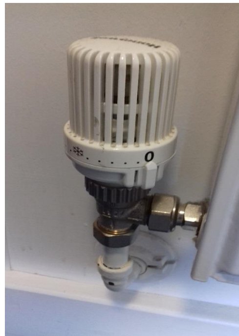
Figure 9 – TRV Off Position
