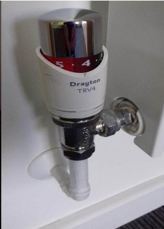
Figure 2 - Radiator Temperature Control (TRV)
