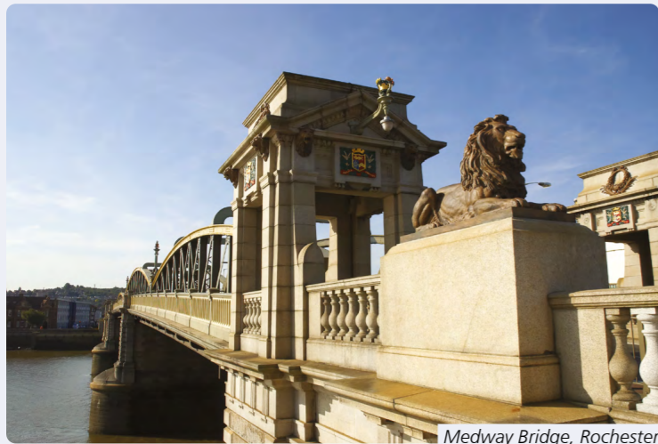
Medway Bridge, Rochester
